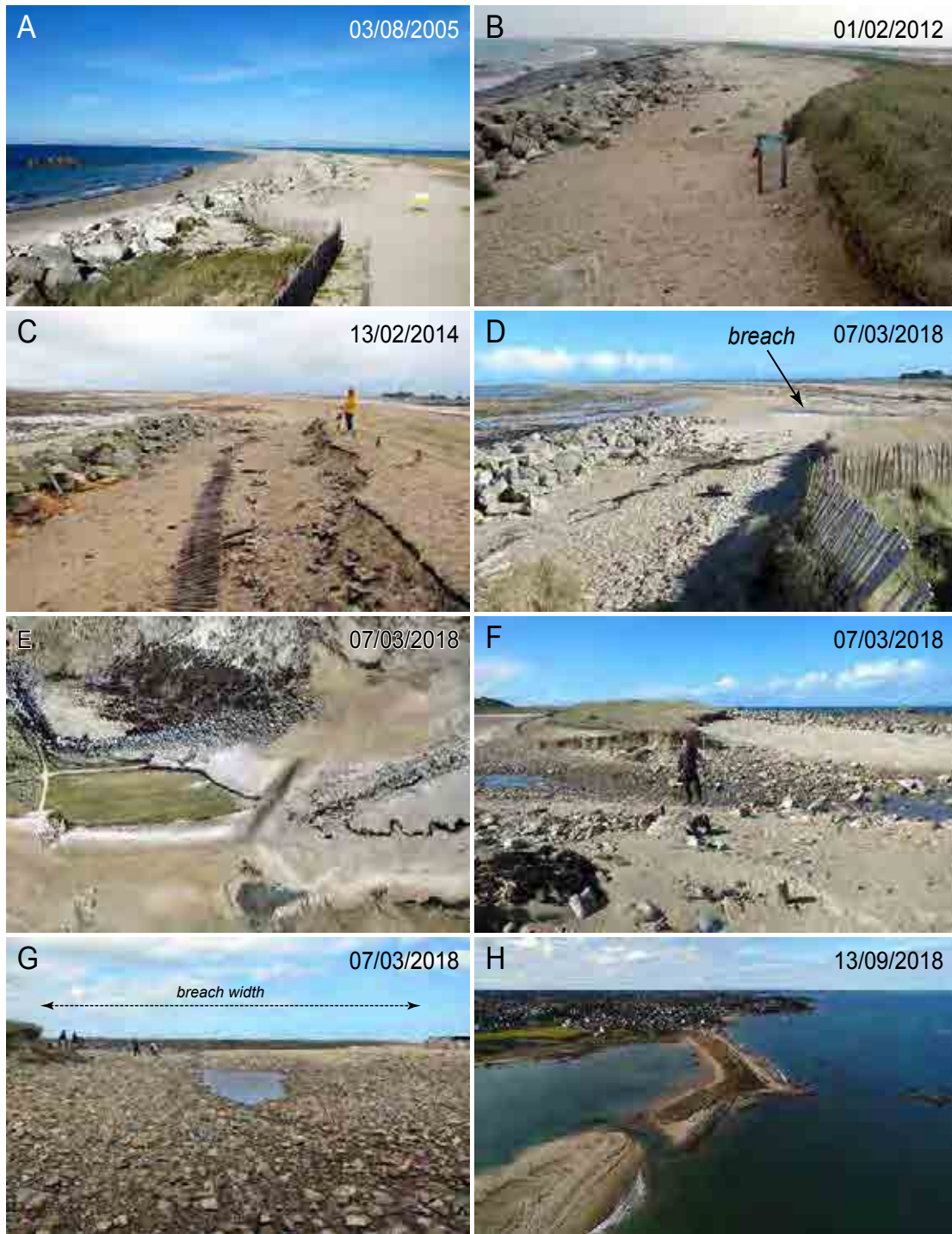
Fig. 13 - Morphological changes of the proximal section situated down-drift of the Chouck groin between 2005 and 2018.
